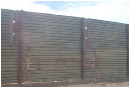
The Wall, Douglas, AZ and Augua Prieta Mexico. Constructed from landing strip materials
